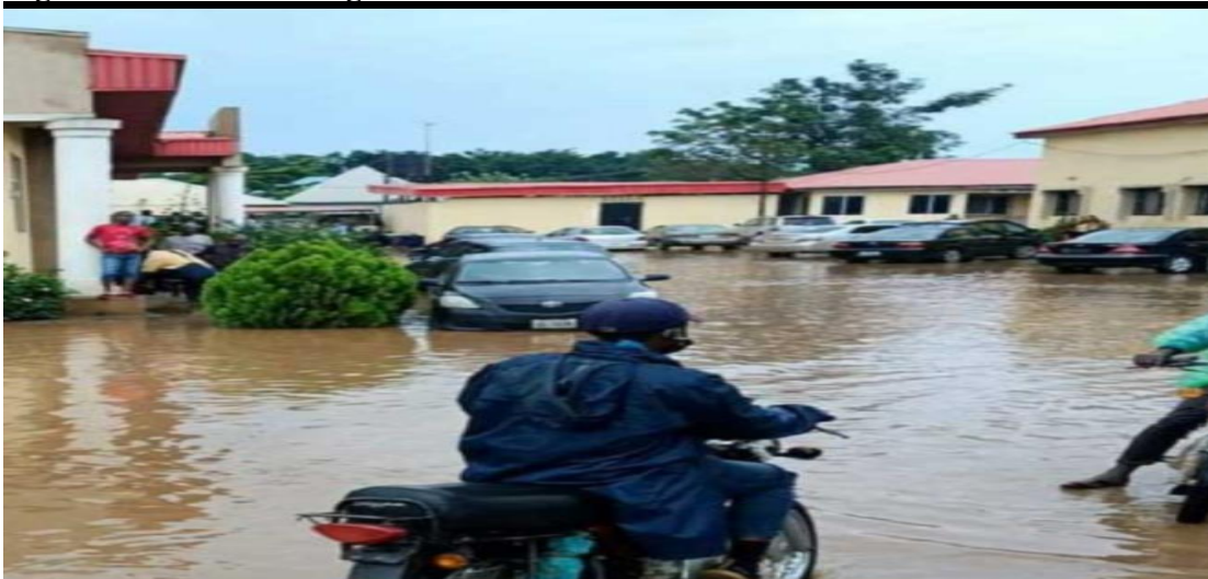
Figure 4: A Flooded High Court in Karu
