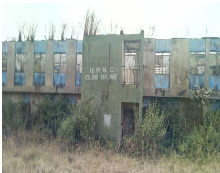
Plate 1: The dilapidated Ugwuoba Progressive Social Club (UPSC) House
